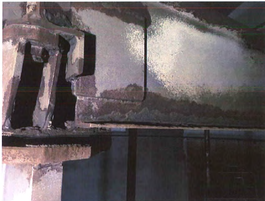
Severely corroded center rafter bearing plate
