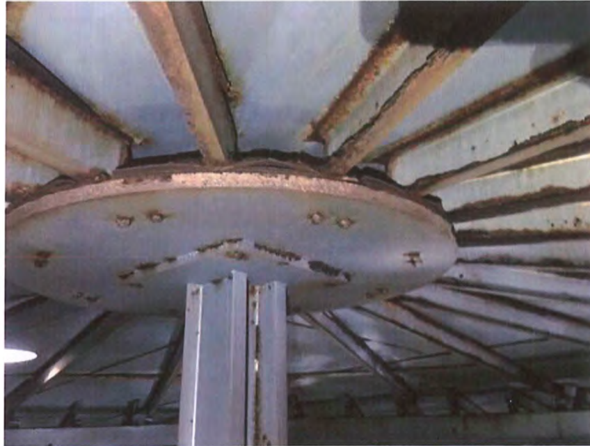
Severely corroded center rafter bearing plate
