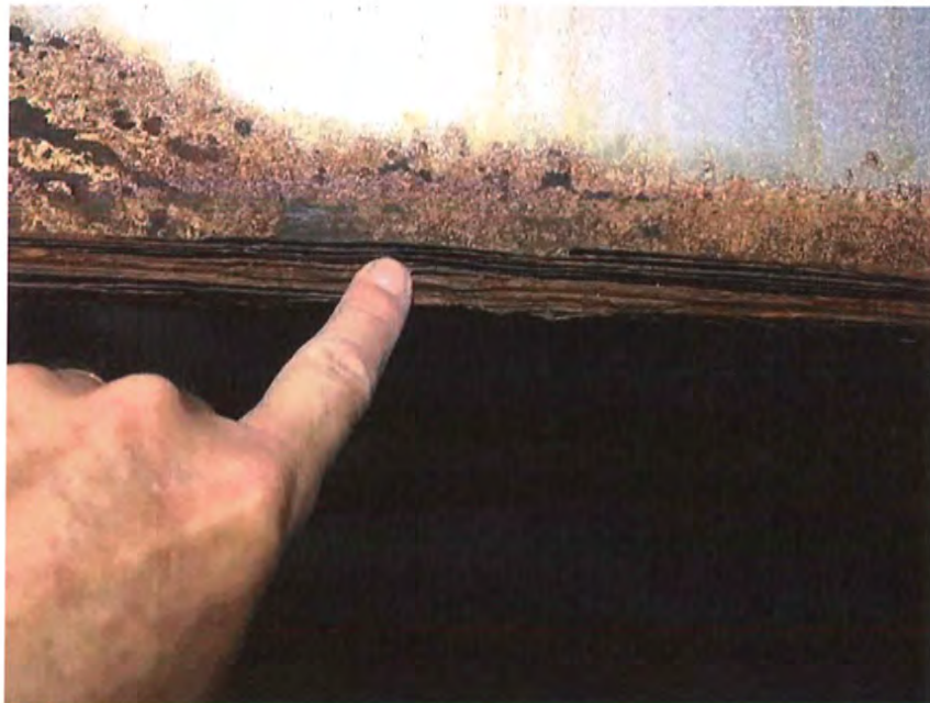
Heavily pitted floor plate near effluent
