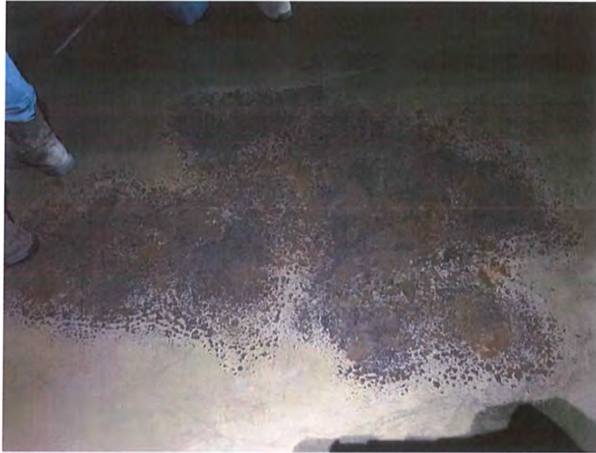
Heavily pitted floor plate near effluent
